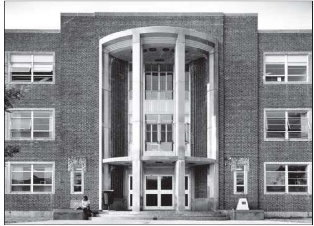
Figure 15. Kingsbury Hall, University of New Hampshire.
