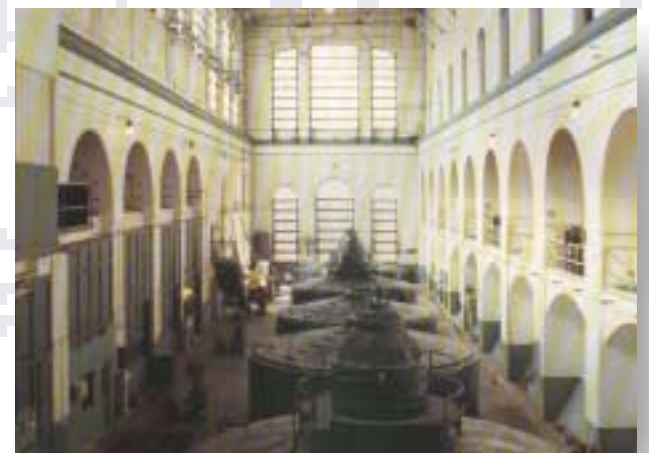
An aerial view of the generators at Holtwood Station, where the first fluid film bearing was installed in 1912.
