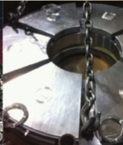
Installation of VK bearing replacement.
