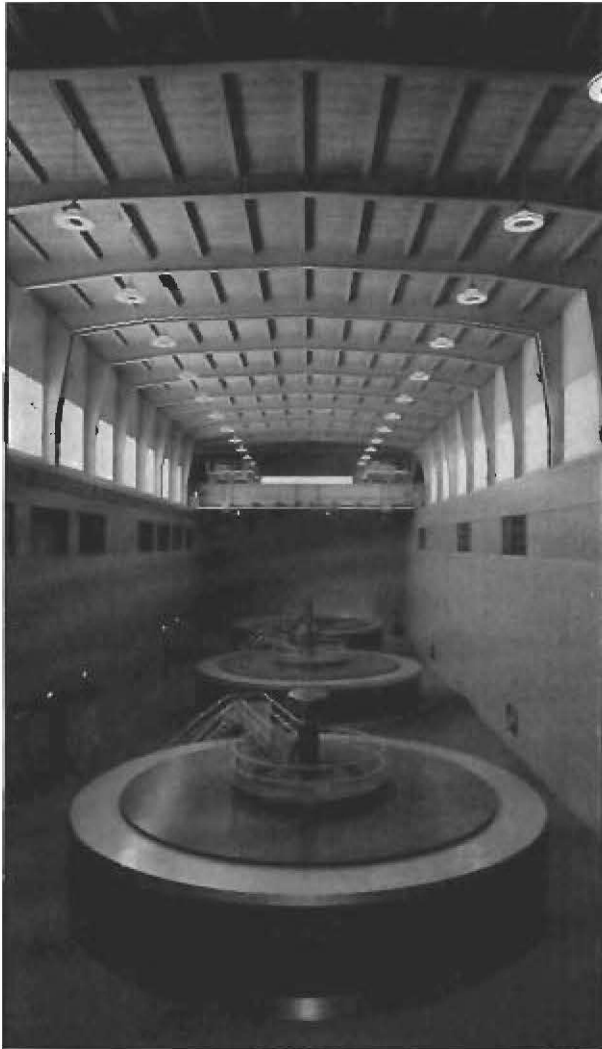
Chickamauga Dam power station, TVA System. Allis-Chalmers generators with Kingsbury 93-in. adjustable bearings. Load 2,075,000 lbs. Speed 75 r.p.m.
