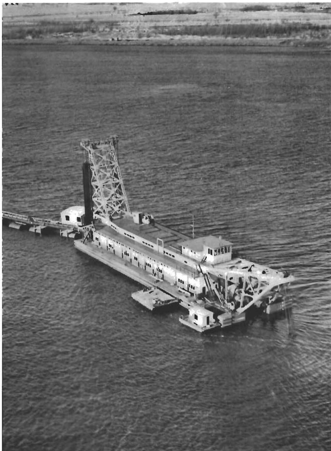
Dredge "Hydro-Quebec" at work on the Beauharnois Canal.
